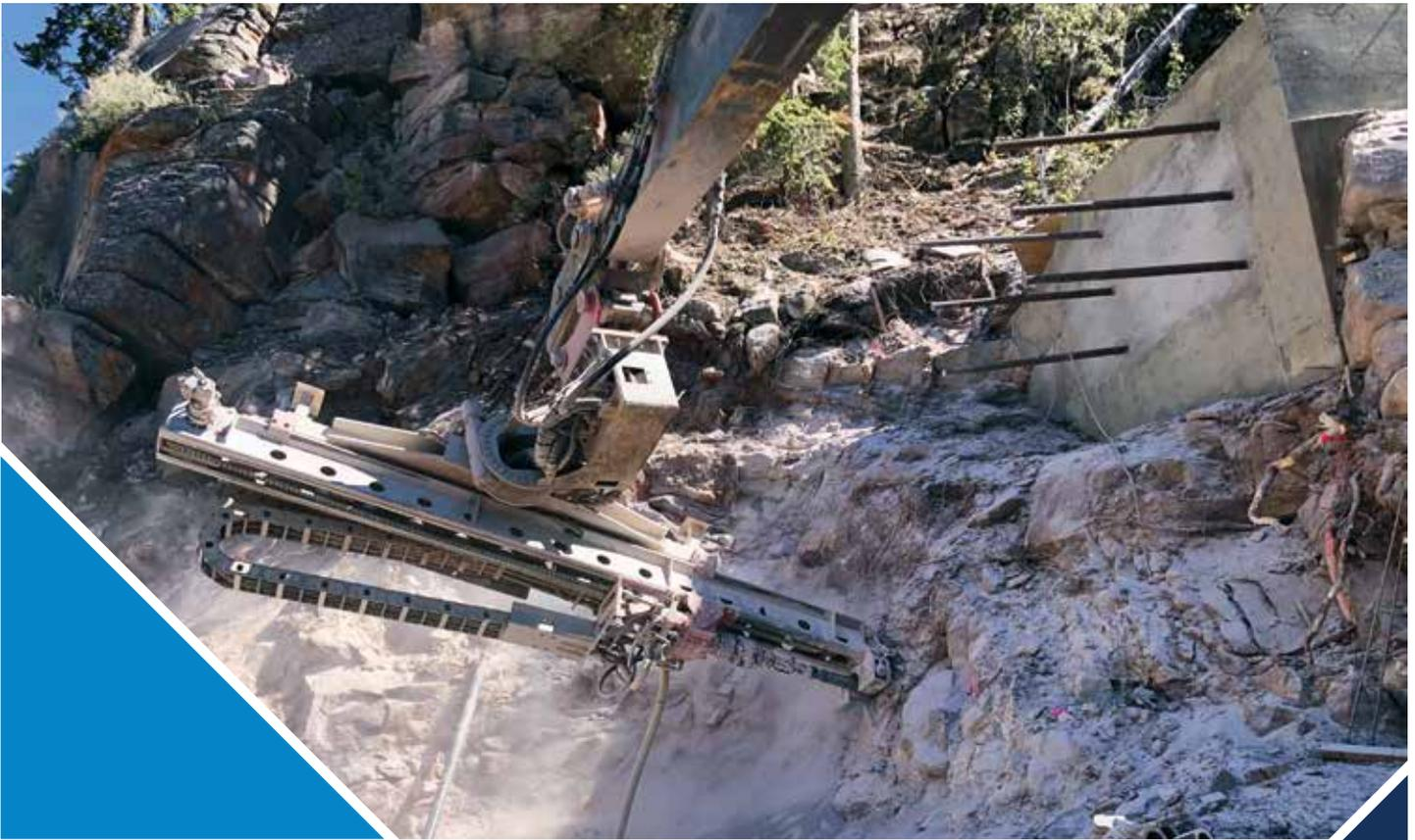
brings the hammer into an idle when the drill string is not fully engaged, and it hangs free when the operator is in a limited access drilling application. The attachment allowed for maximum performance and operation in the tightest, most extreme conditions.
